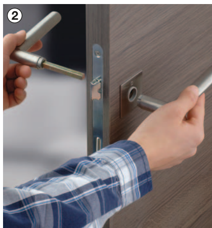
2 Put the door handles together
