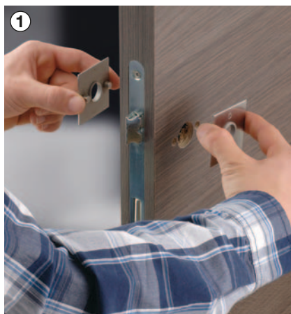
1 Place the roses in position
